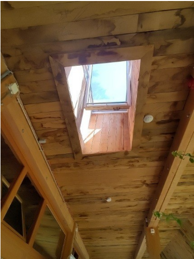
Roof opening, EuroSolar photograph [E, p. 8].
